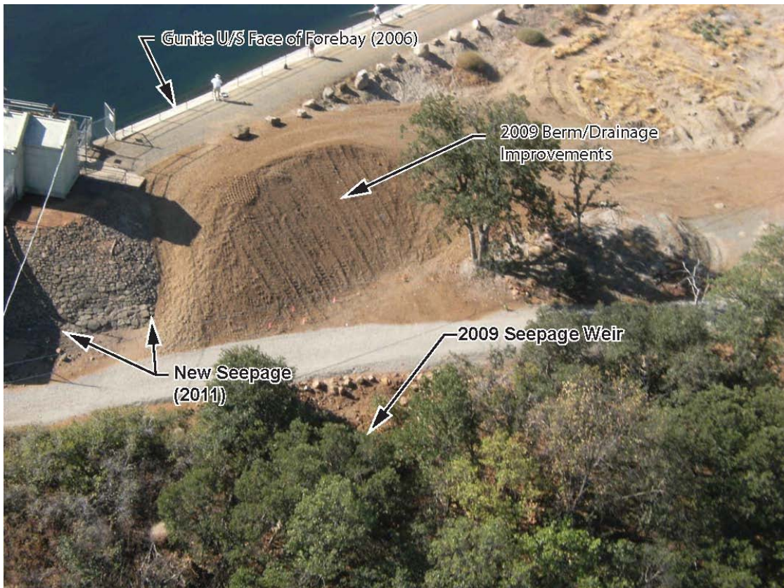
Figure 12. Aerial View of Hat Creek Forebay Embankment Showing History of Repairs.
