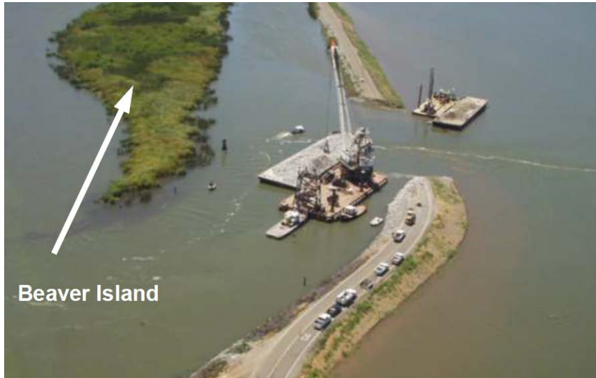
Figure 4. Levee Breach along Middle River in Upper Jones Tract.
