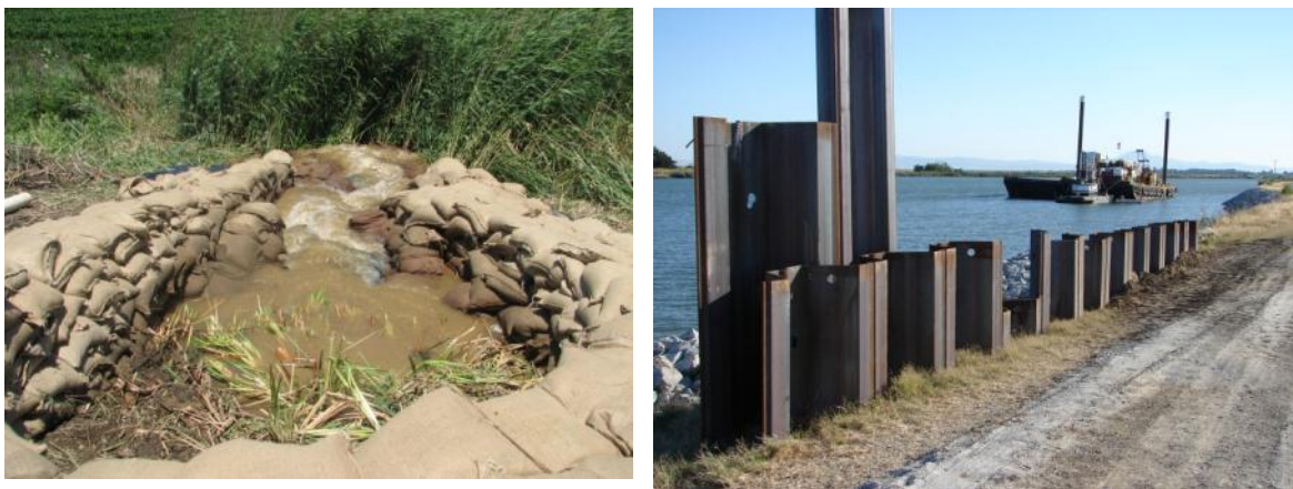
Figure 11. Sand Bag Ring Around Landside Boil and Sheet Pile Wall along Staten Island Levee to Prevent Near Breach.
