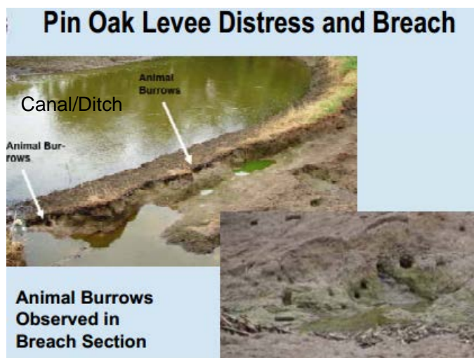
Figure 8. Levee Breach along Pin Oak Levee System.
