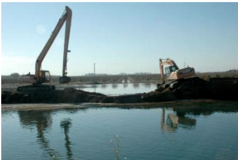
Figure 6. Levee Breach along Glenn-Colusa Canal near Ord Bend.
